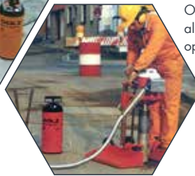
Drilling out water valves (Ø 200 mm / 8")
