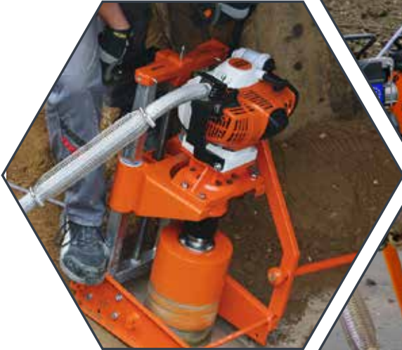
90° drill in sewage pipe. Pipe base clamped between concrete pipe and trench and secured by ground spikes.
